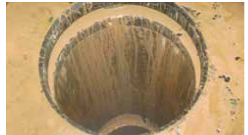
BOP cavity free from metal debris.
