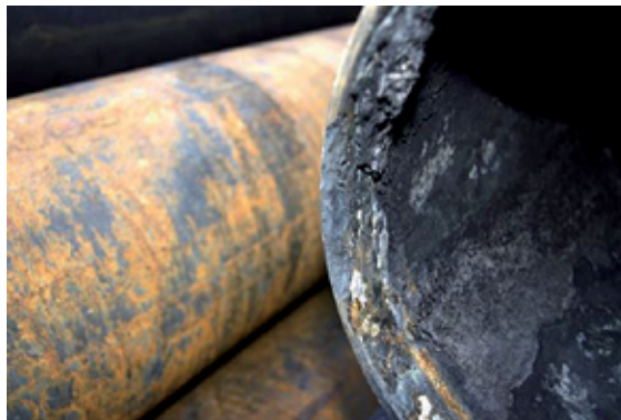
Picture of severe localized corrosion on the pin end of the 10 3/4" tubing.
