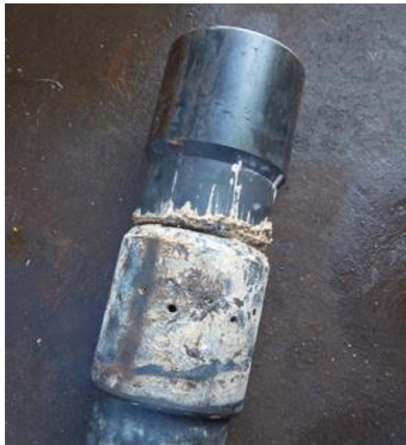
Scale at the top of lock
